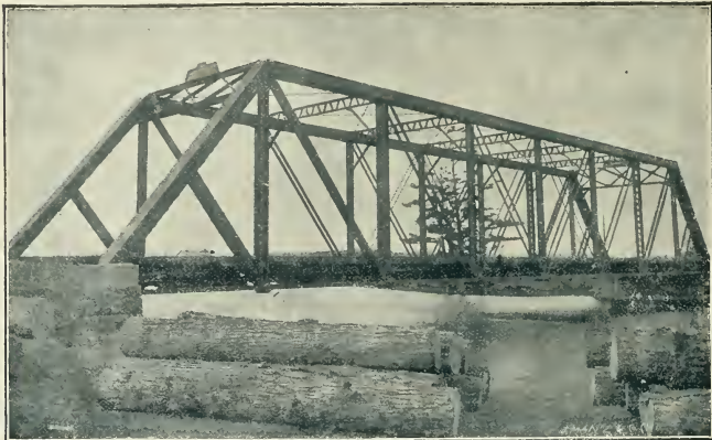
1-192 x 30 FEET. STEEL SPAN.
